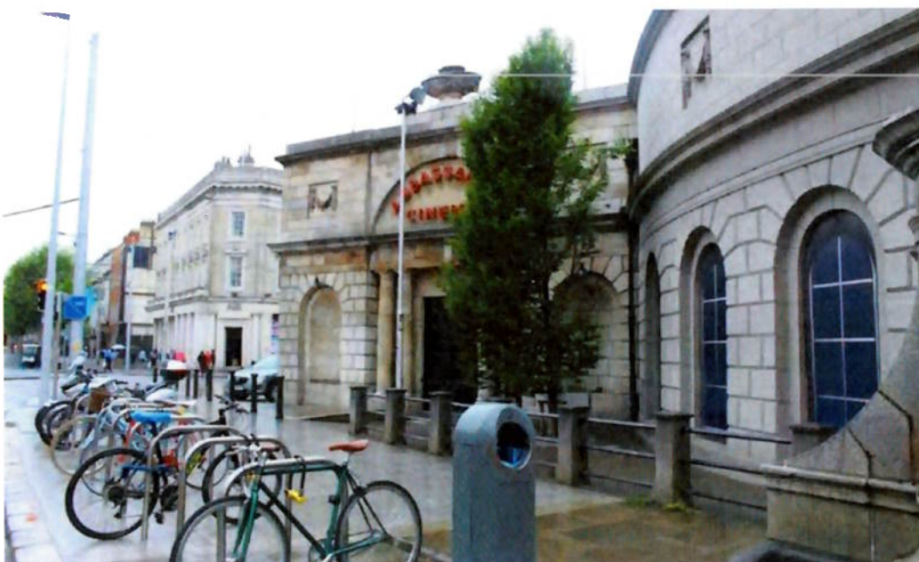
Figure 19 View of East elevation both granite and rendered facades
