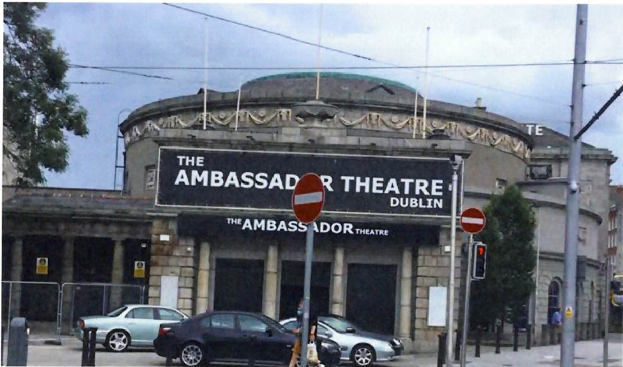
Figure 1. External Elevation of the Ambassador Cinema.
