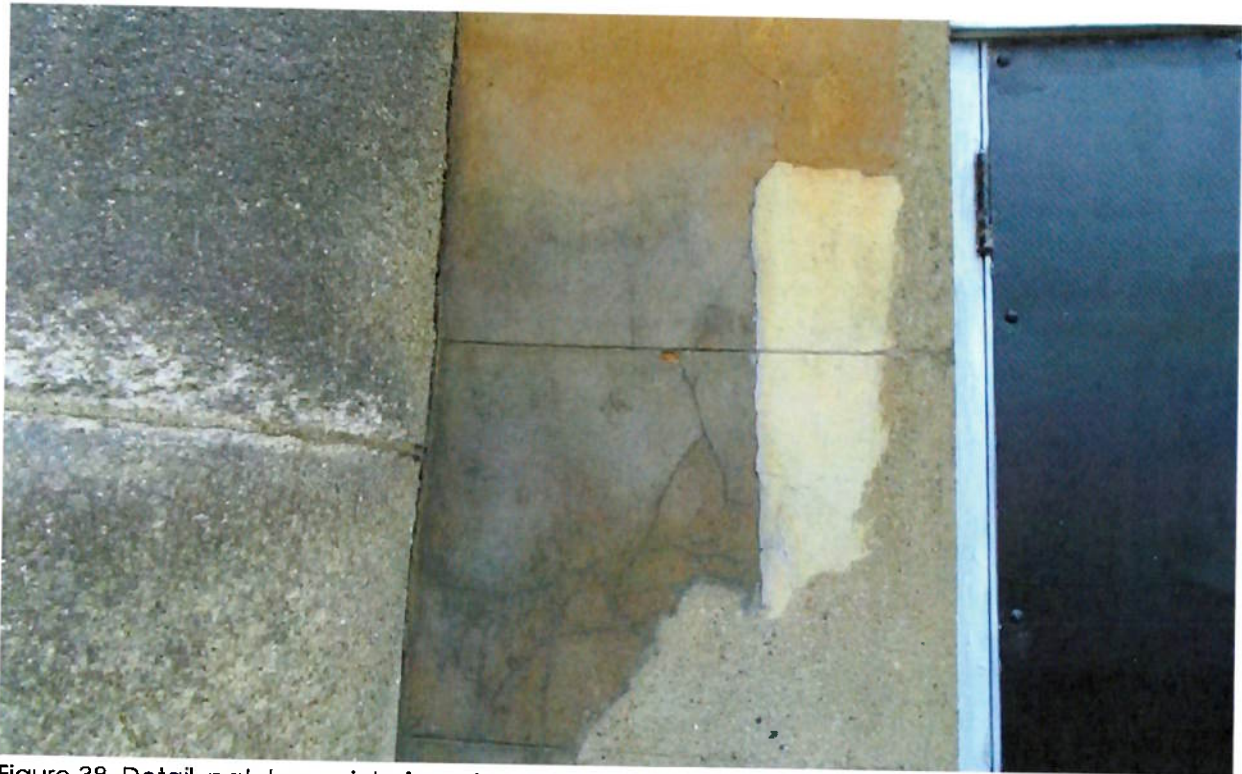
Figure 38. Detail, patch repair to facade
