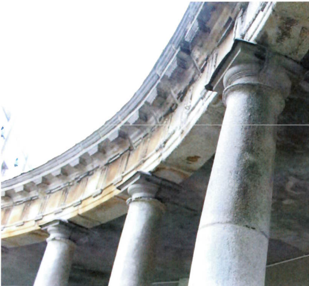
Figure 19. View of upper cornice to the arcade.
