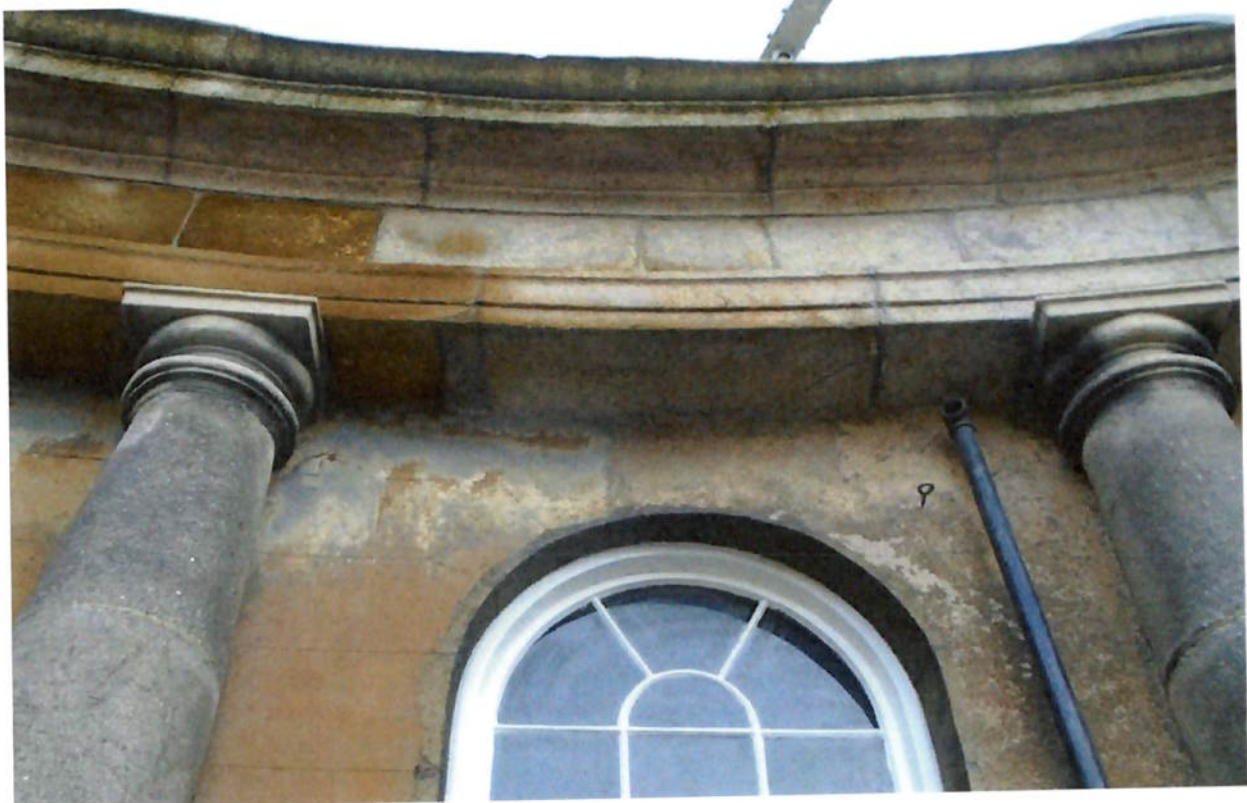
Figure 37. Note, concrete replacement capitals
