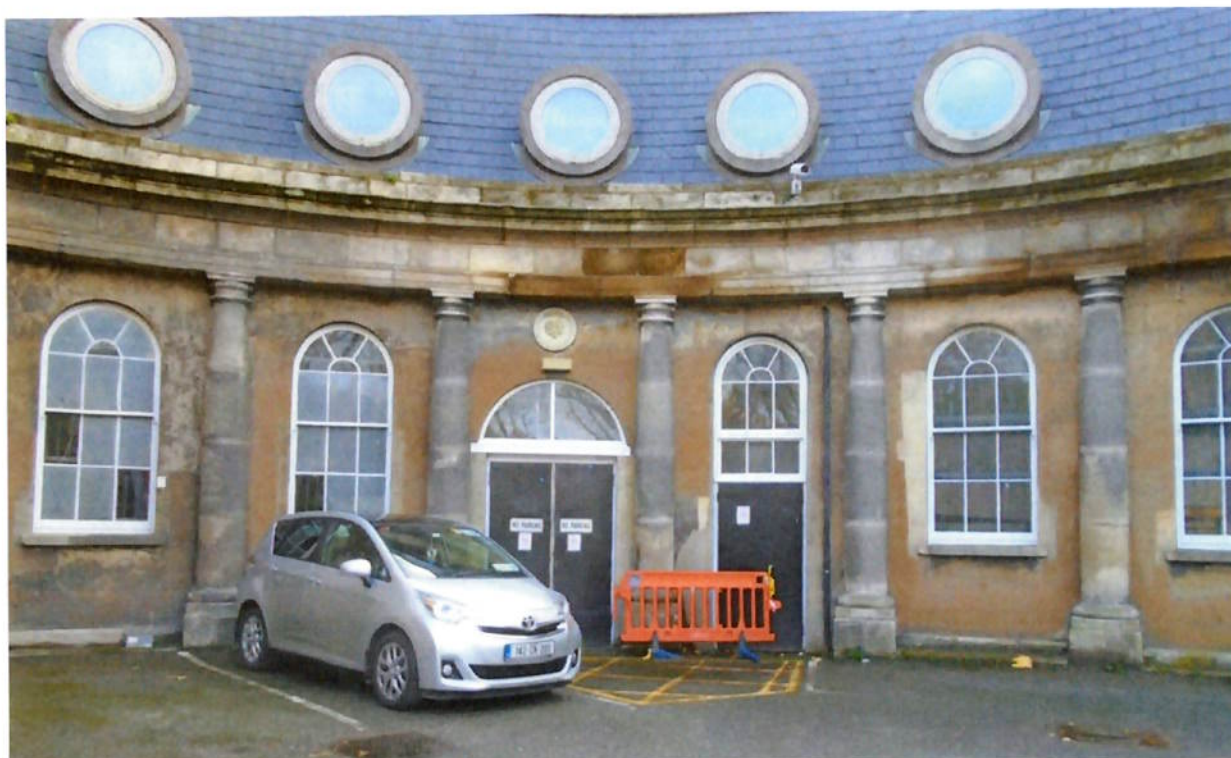
Figure 28. Rear elevation facing into courtyard
