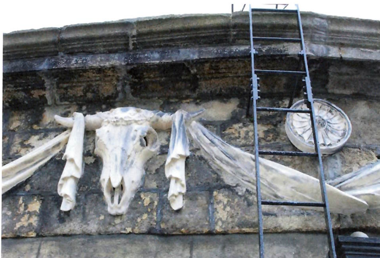
Figure 6. Replaced 'new' Coade Stone elements.
