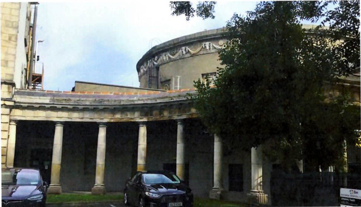
Figure 3. External Elevation of the Ambassador Cinema.
