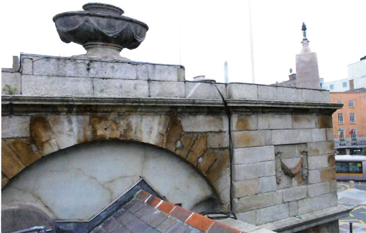
Figure 16. Upper level of the return elevation.
